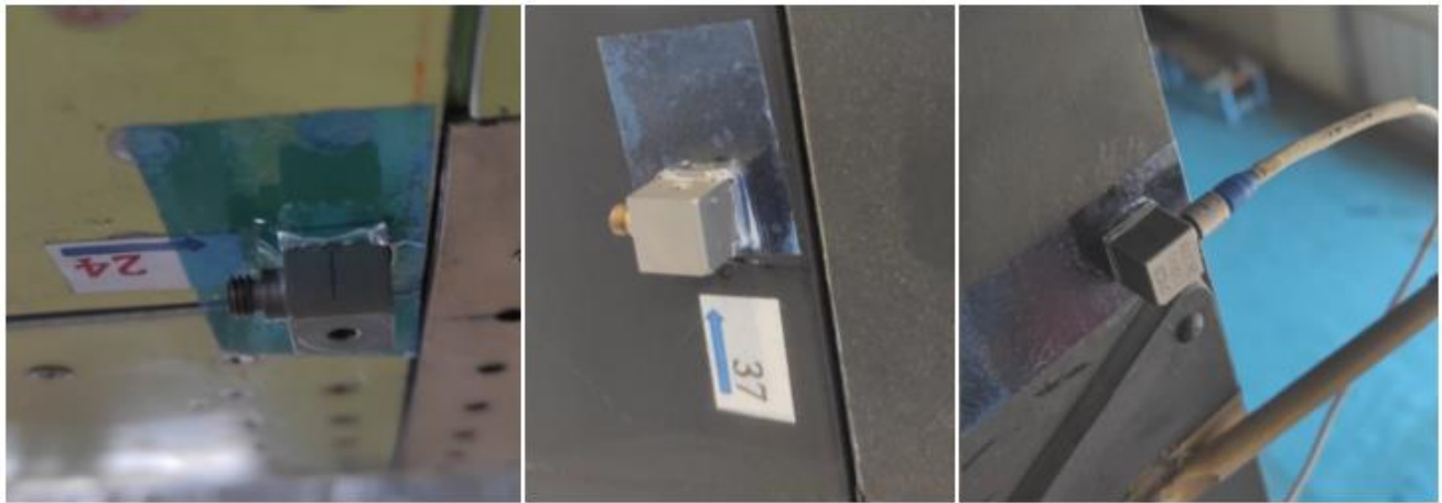
Figure 12 – Examples of accelerometers installation
